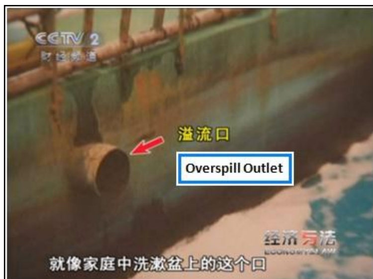
Figure 3: Overspill outlet adjusted over the pool
